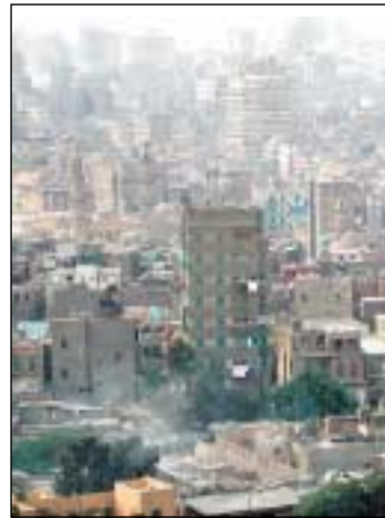
Urban buildings in Cairo
